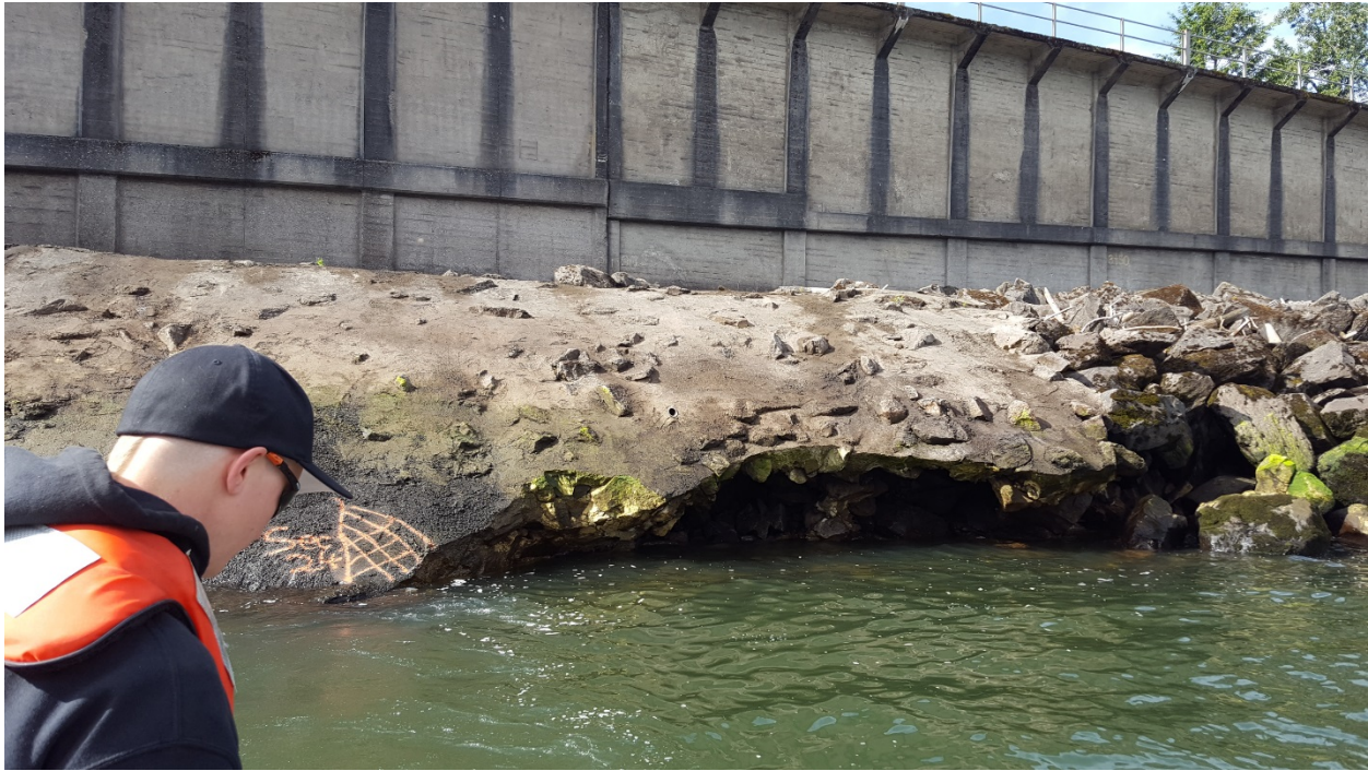
Figure 3-6: Bonneville B-Branch Fish Ladder Downstream Erosion at Section 24 Looking South
