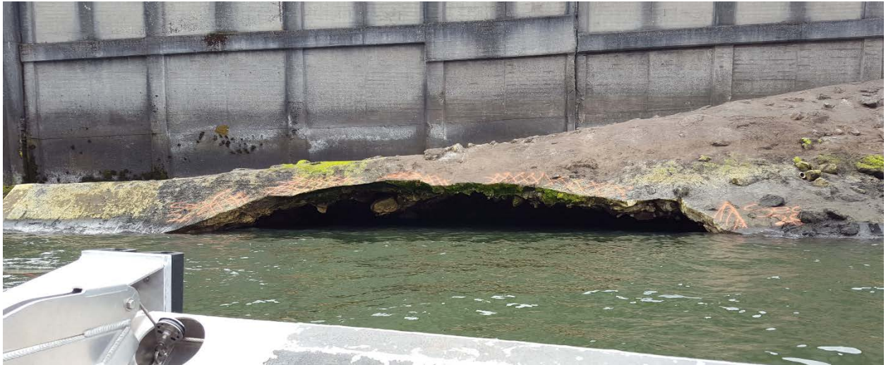
Figure 3-3: Bonneville B-Branch Fish Ladder at Section 25-26 Looking South
